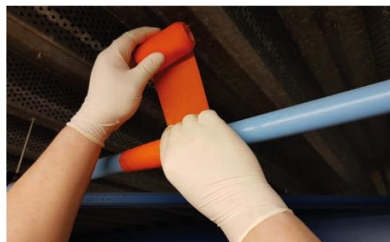
PipeRepair being applied
