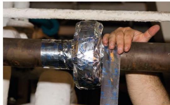
SprayStop being applied
