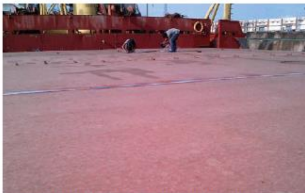
HatchCover tape being applied on a vessel
