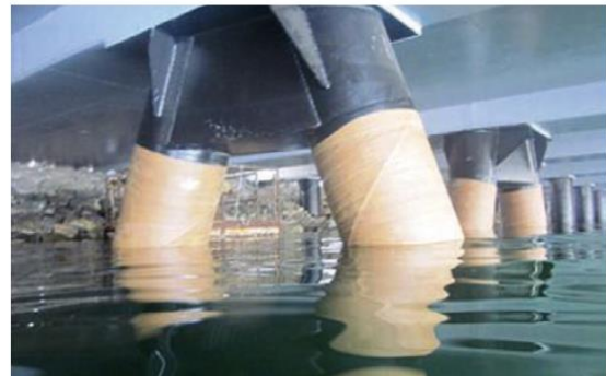
RustStop applied underneath a bridge
