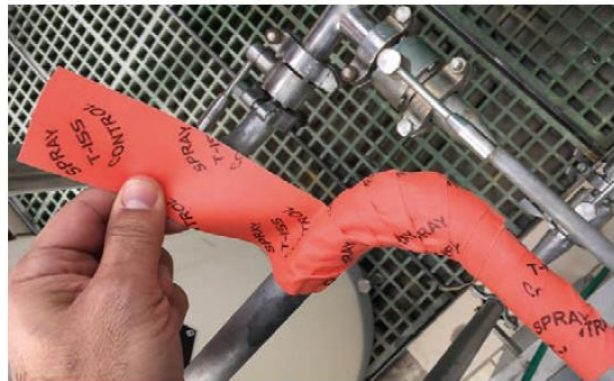
SprayControl being applied
